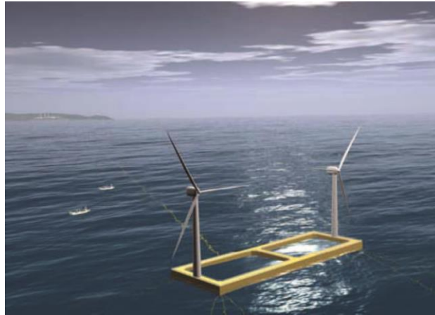
Figure 1.14 Prof Ohta's concept of pontoon-type wind turbine with rotor shroud nozzle (Wang, 2010)
