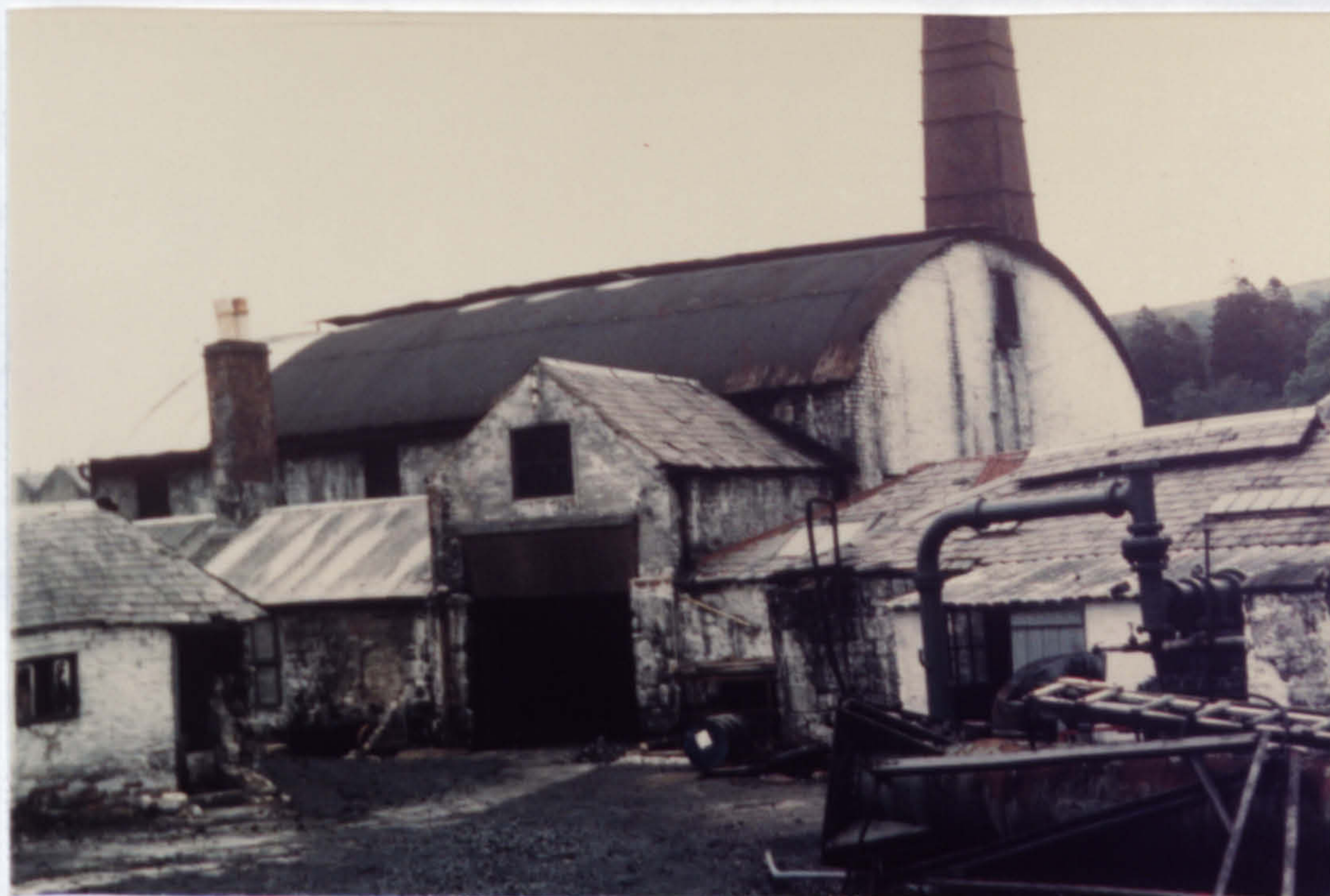
Horizontal-retort house at Langholm (1973). Typical spacious design capable of storing coal or spare retorts if necessary; surrounded by outhouses - tool store on left, purifier sheds and governor house on right.
