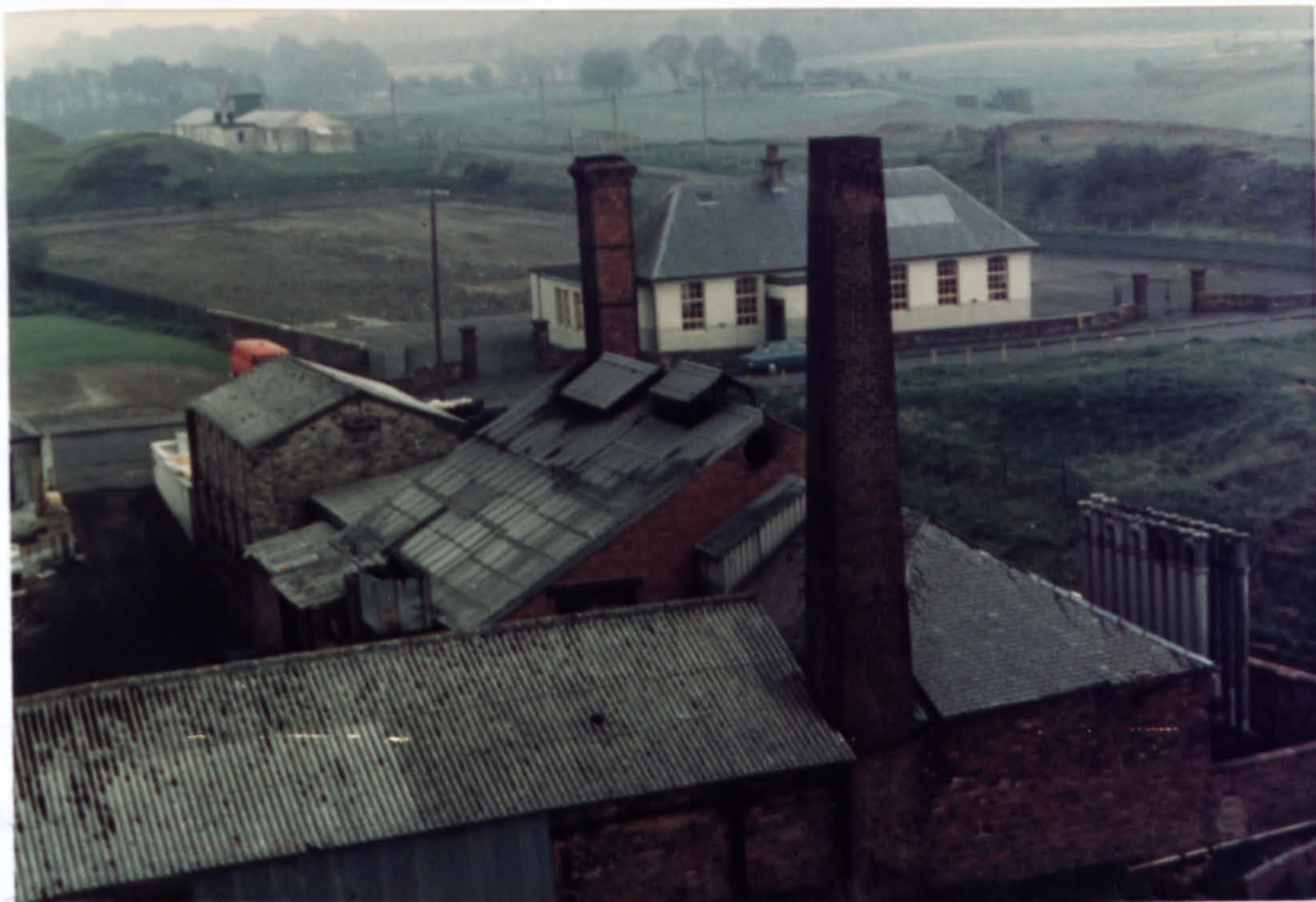
Fig. 3.17 Horizontal Retorts and Retort House at Muirkirk (1973)
