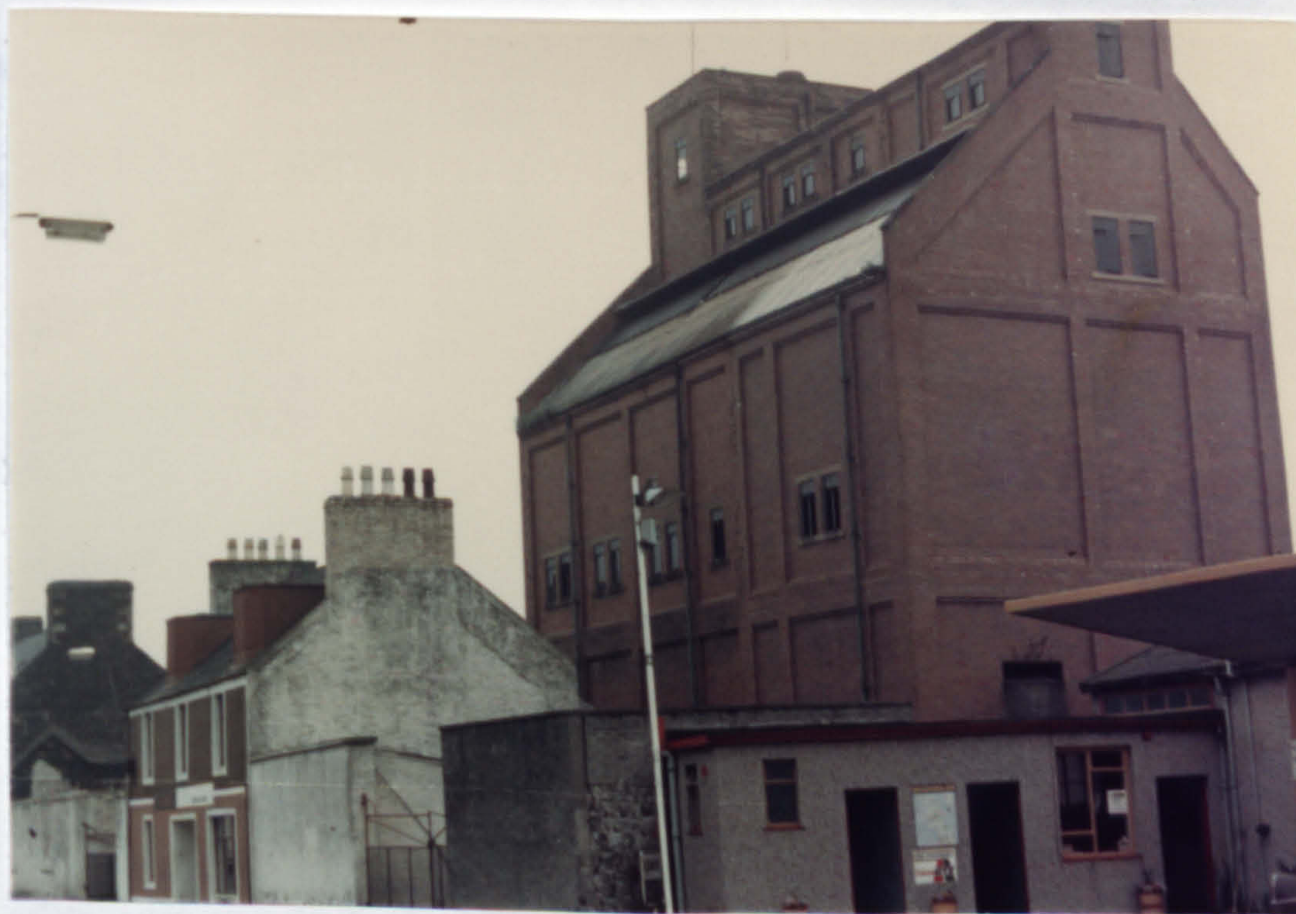
Small vertical-retort house at Stranraer (1974). Tall building closely tailored to internal machinery. Typical rectangular projection on left gable at summit of mechanical elevator feeding horizontal conveyors to coke hoppers. Note use of adjoining dwelling house as gas appliances showroom.
