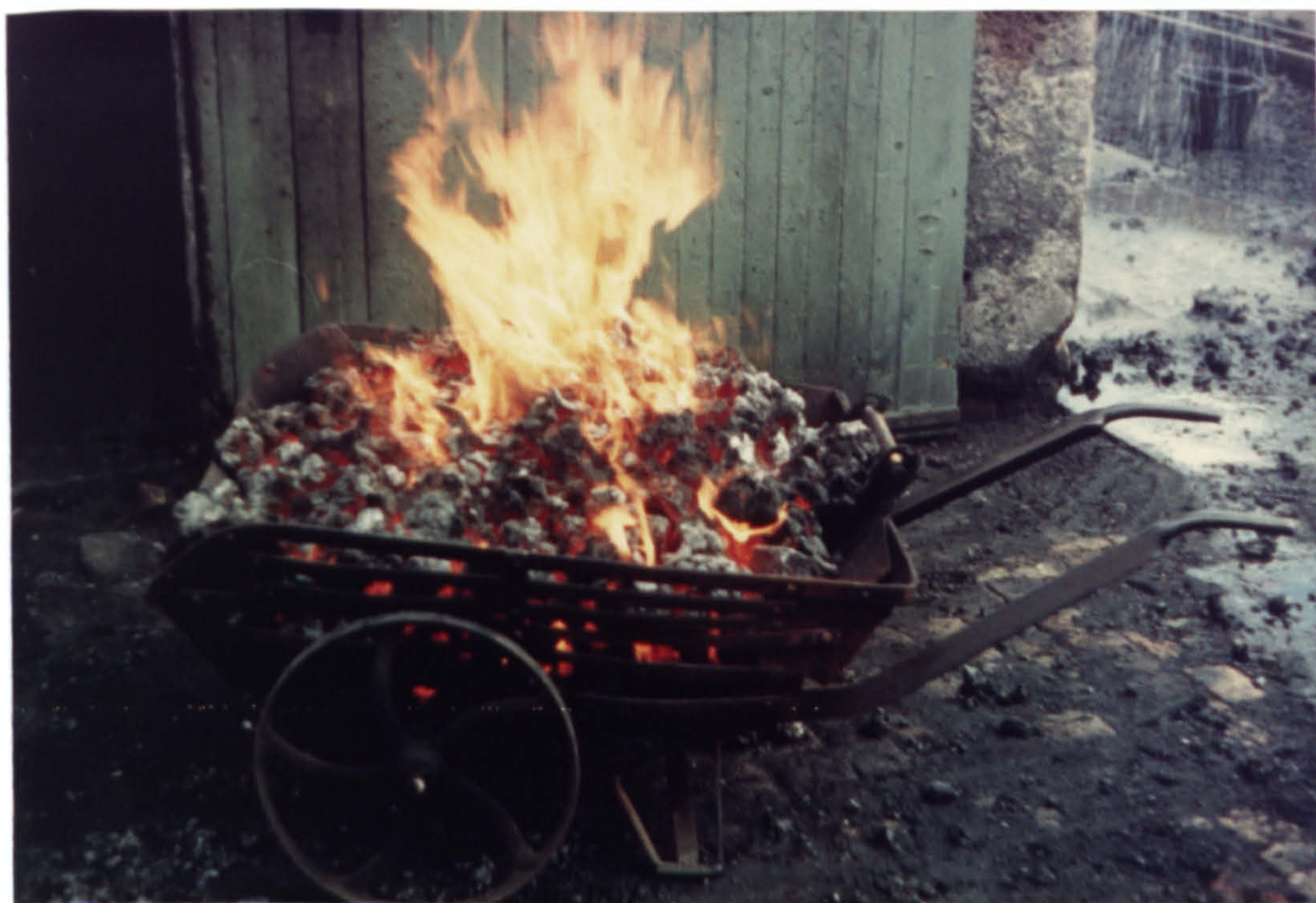
Fig. 3.30 Quenching Coke at Biggar Gasworks (1972)
