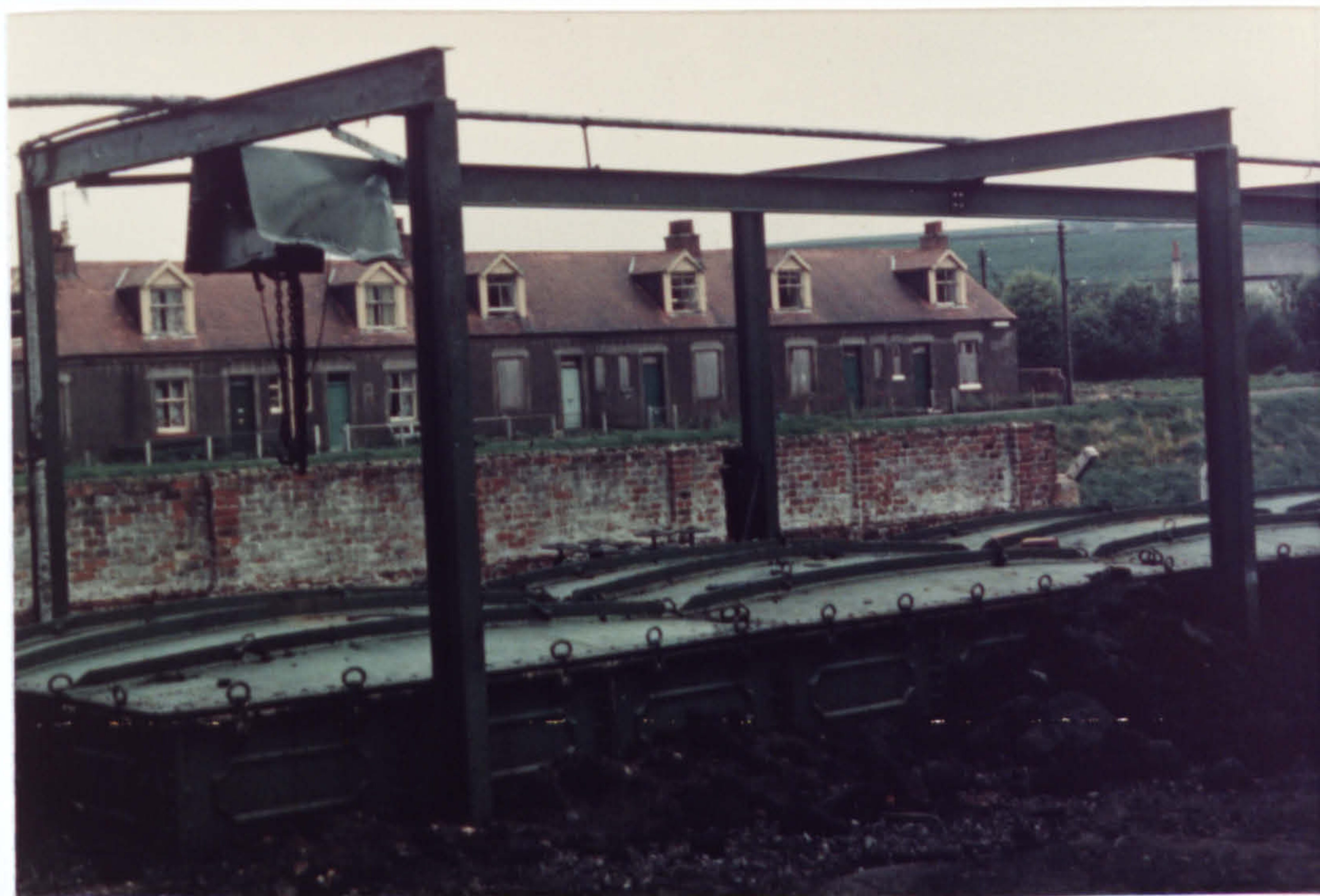
Fig. 3.53 Purifiers at Kirkconnel (1973) and Edinburgh (1972)
