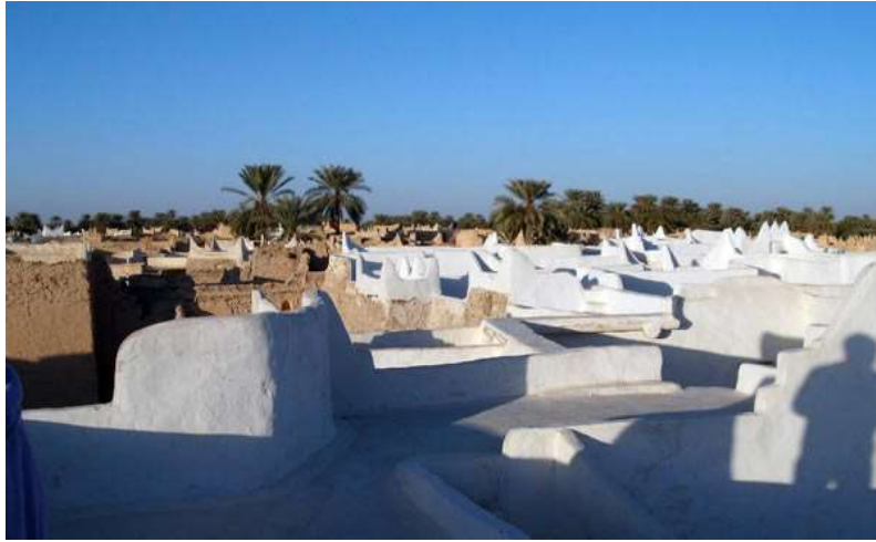
Figure 2.2: In Ghadames Women use Special Streets Built above the Roof. Source: Temehu.
