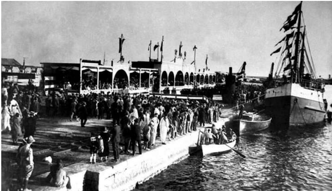
Figure 6.1: An Old Image of Benghazi harbour. Source: Tours libya.com.
