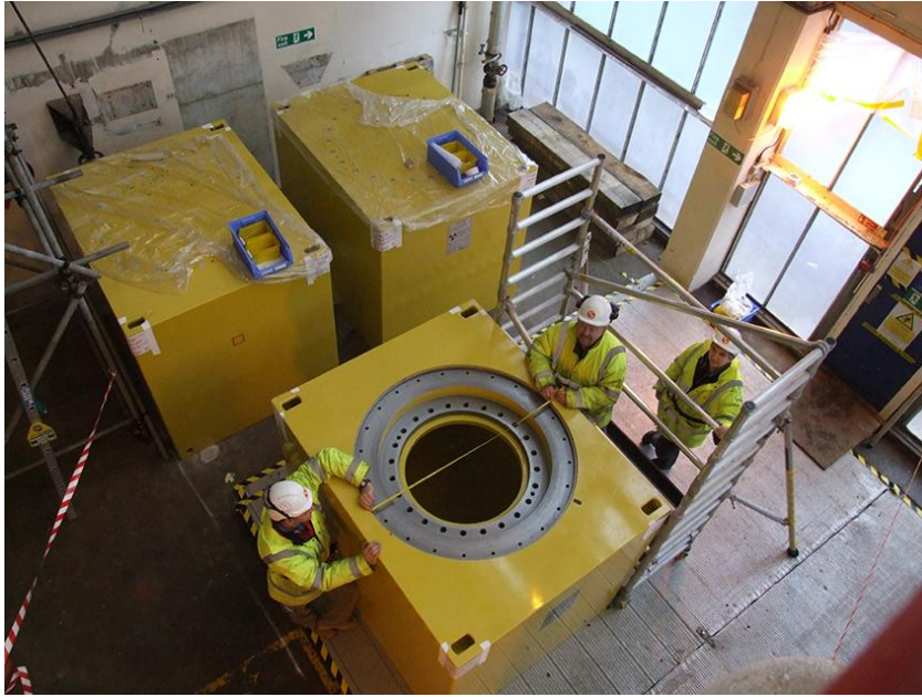
Figure 2-20 Thick walled DCIC self-shielding Mini-Stores at Dungeness A power station (Courtesy of NDA)
