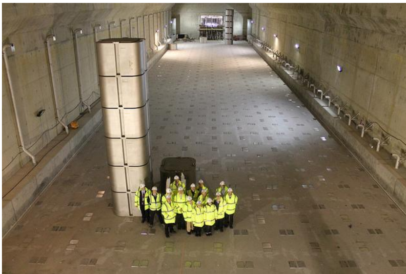
Figure 2-19 Hunterston A stacking of demonstration ‘single use’ unshielded 3m 3 stainless steel boxes for ILW in their shielded long term-interim stores (Courtesy of Magnox Sites)
