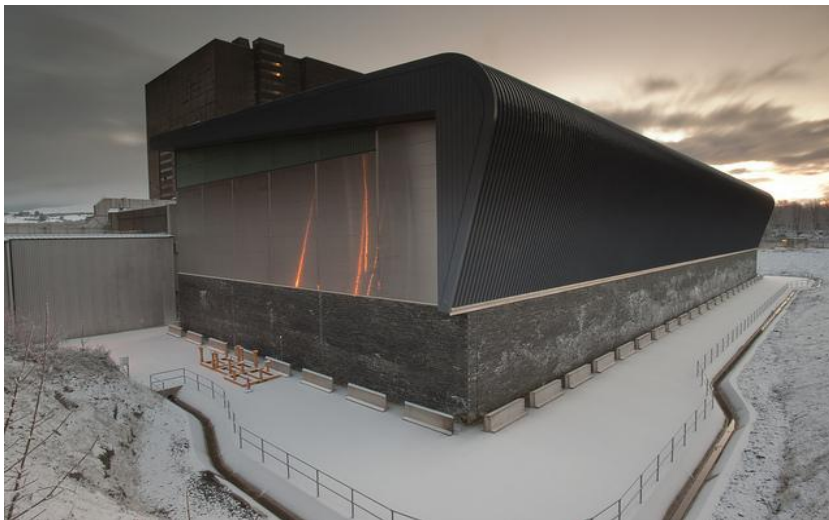
Figure 2-17 Trawsfynydd unshielded long-term interim store (Courtesy of Magnox Sites)
