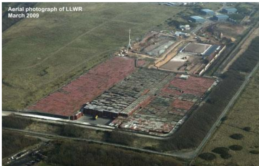
Figure 2-5 Low Level Waste Repository near Drigg in Cumbria showing the current disposal vaults and grouted ISO freight waste containers in the foreground (reproduced from NDA website)
