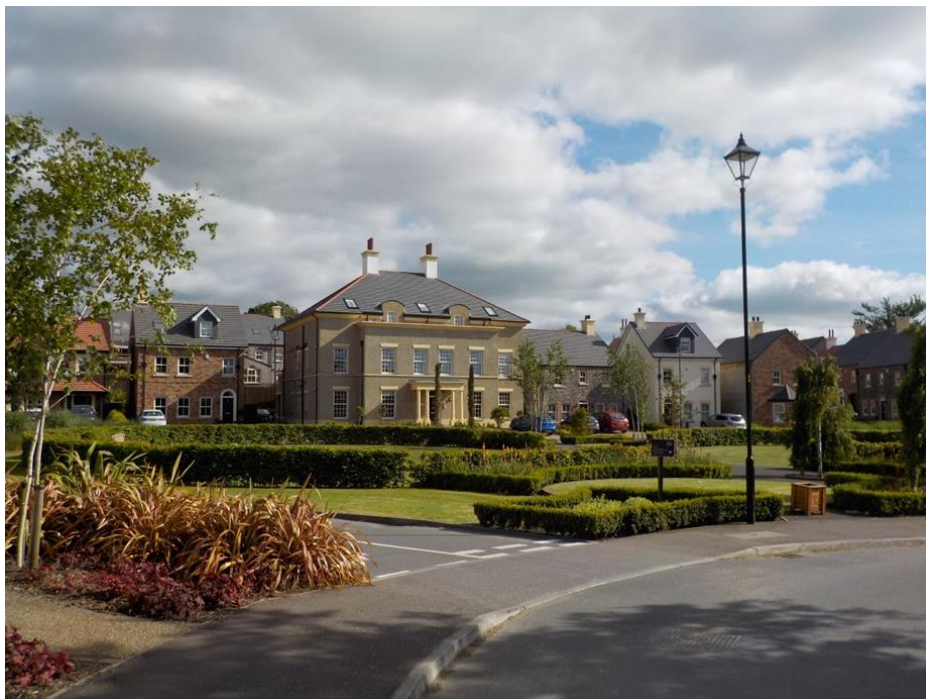
Figure 25: Hawksmore House: A housing with care prototype
