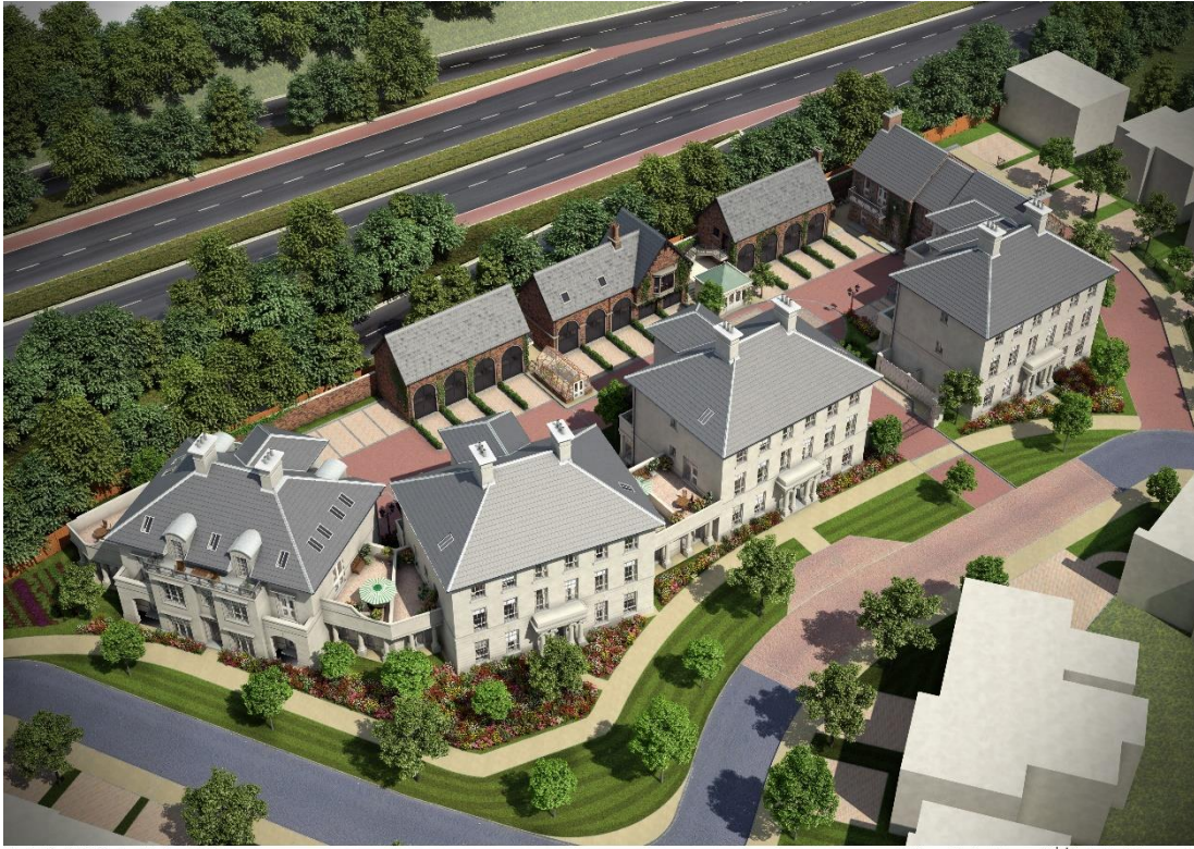
Figure 63: The Pavilions: A proposal for 27 Extra Care dwellings with supporting facilities and community navigator.
