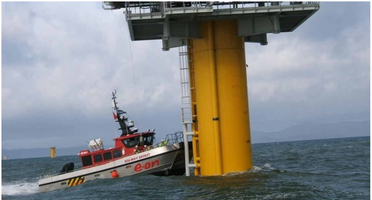
Figure 4.24: Crew transfer to a mono-pile foundation wind turbine from sea
