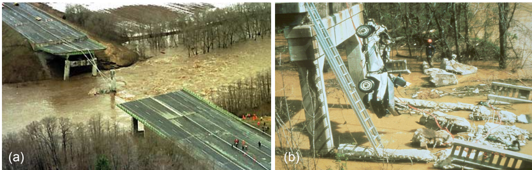
Figure 2.3: (a) The Schoharie Creek Bridge collapse due to severe foundation scour with 10 fatalities, source: AP (1987 cited in UMKC, n.d.). (b) The impact of the Hatchie river road bridge with 8 victims, source: Briaud, (2011).
