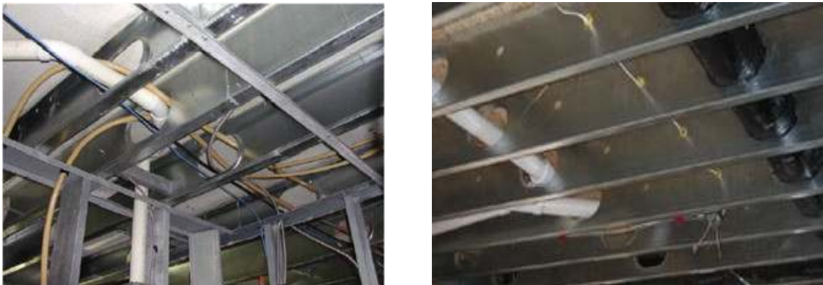
Figure 1.1 Cold-formed steel with web holes
