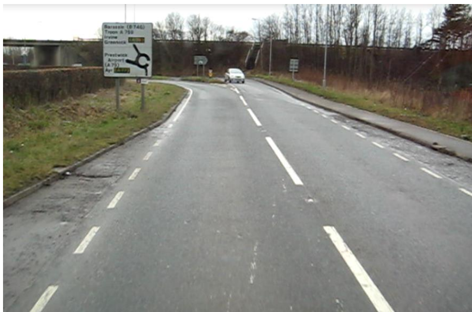
Figure 3-12 - Hard Braking Manoeuvre on Approach to Roundabout
