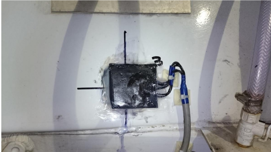
Figure 3-8 - Strain Gauge Rosette No.3 – Covered
