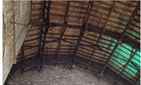
Figure 129: The roof of Tron Church in Edinburgh (1636-48)
