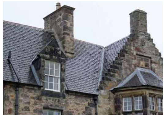
Figure 187: Slate roof at Pinkie House (1613)
