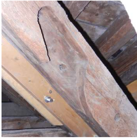
Figure 170: Redundant lapped/halved joints found in Blair Castle (1745)
