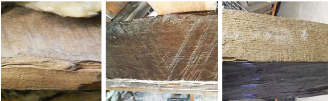
Figure 192: Saw marks on collars in King's Old Buildings at Stirling Castle (1557) (left), collars in Kelburn Castle (1581) (centre), struts in Newhailes House (1733-51) (right)
