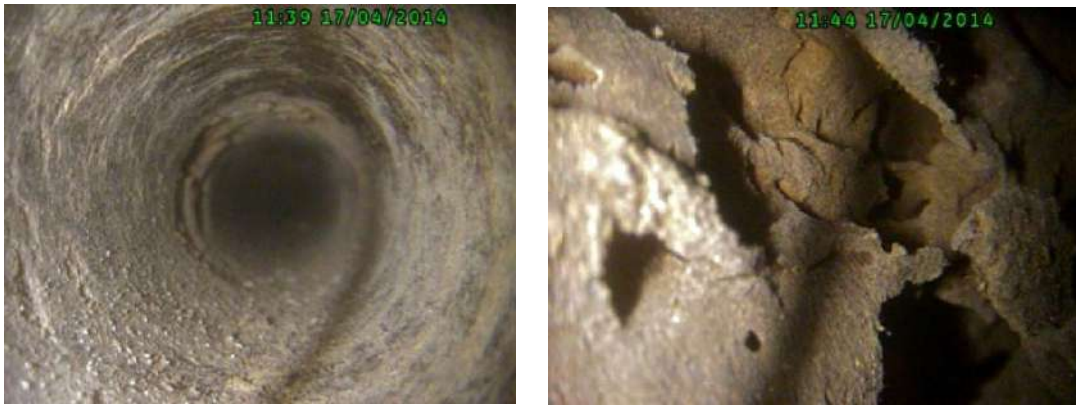
Figure 23: Example of pictures taken with an endoscope inside a borehole in a timber strut (Kloiber et al., 2015a)
