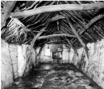
Figure 111: Cruck-framed Cottage in Torthorwald (RCAHMS SC 383456, 1970)
