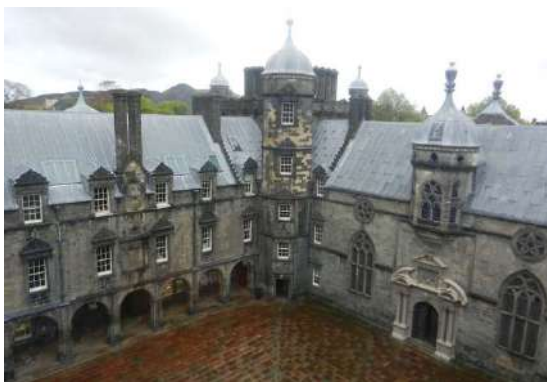
Figure 188: Lead roofs at George Heriot's Hospital (1633-37)
