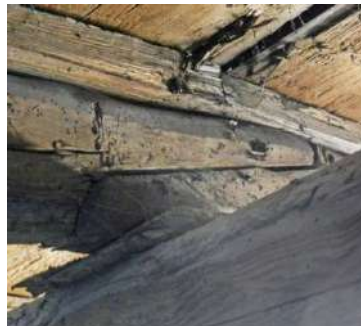
p) Kinross House (1679-93): scarf joint secured by metal nail (upper beams)
