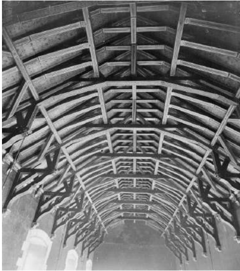
Figure 109: The roof of the Great Hall at Edinburgh Castle (1510) (RCAHMS SC 1201162, 1888)
