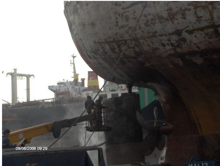
Figure4.18. Good surface cleaning done by 2500 bar water pressure
