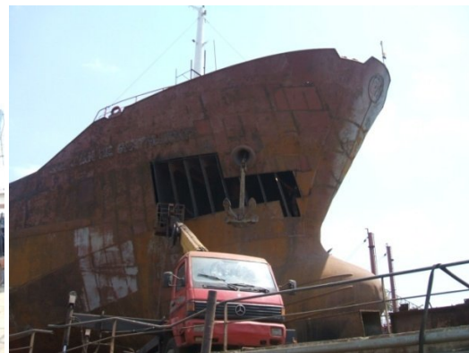
Figure 4.4. Front shell plate steel replacement
