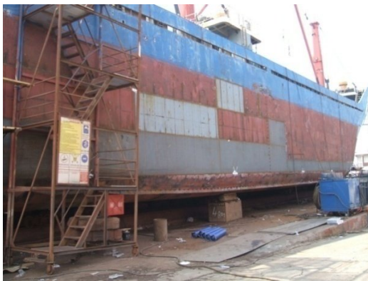
Figure4.3. Shell plate steel replacement
