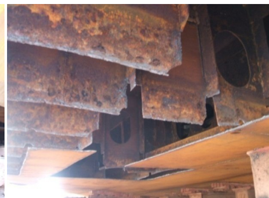
Figure 4.6. Double bottom repair work II
