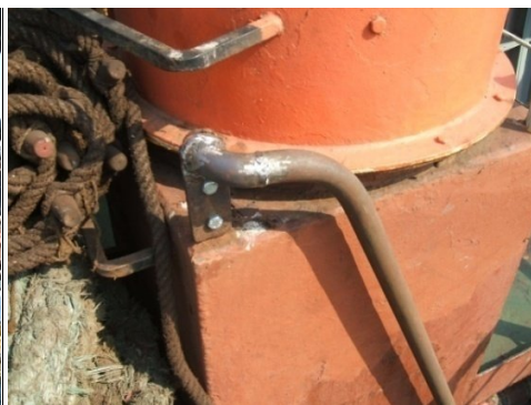
Figure4.9.b New ladder handle
