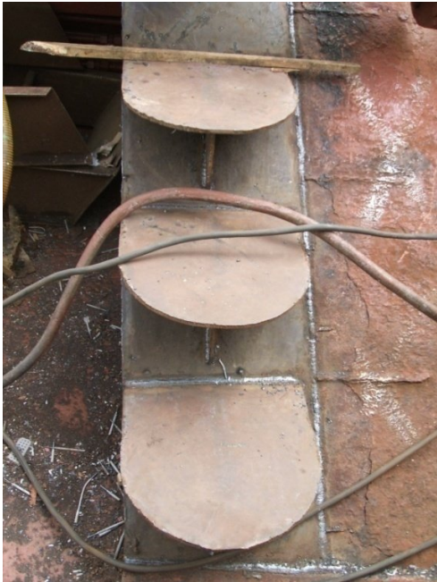
Figure 4.7.b. New ladder sample
