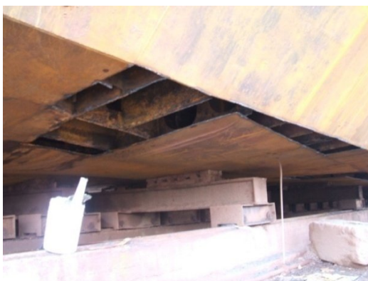
Figure4.5. Double bottom repair work
