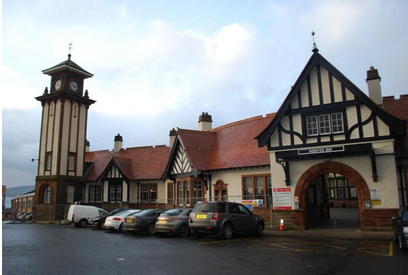
Figure 6-2 Refurbished Exterior at Wemyss Bay
